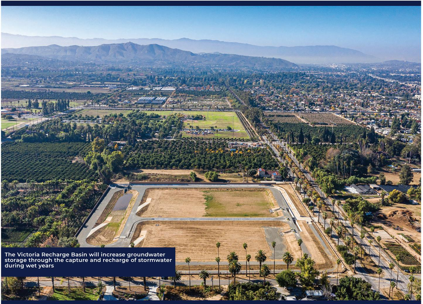
The Victoria Recharge Basin will increase groundwater storage through the capture and recharge of stormwater during wet years
