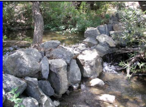
50 Arroyo Chub were released at this grade stabilizer after water quality improvements were made to Sycamore Creek.
